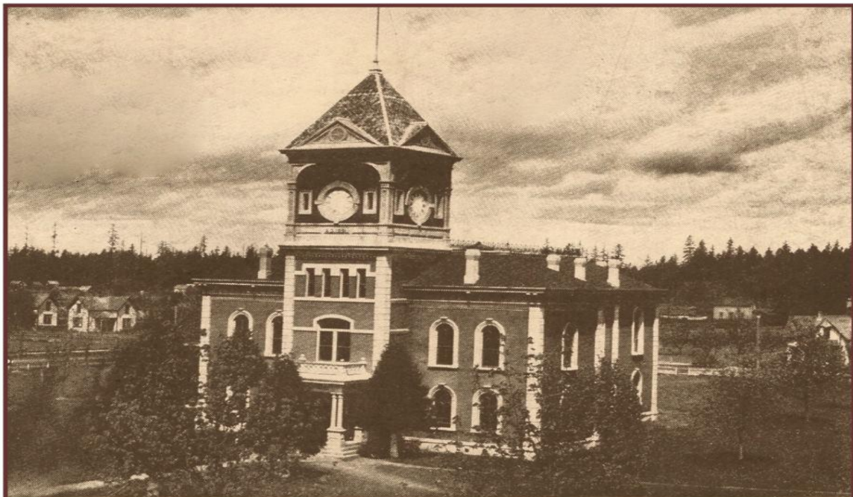
5001 WASHINGTON COUNTY COURT HOUSE. HILLSBORO. OREGON
